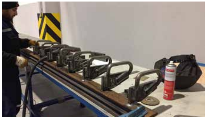
Anchorage Welding of AR-EX HS
