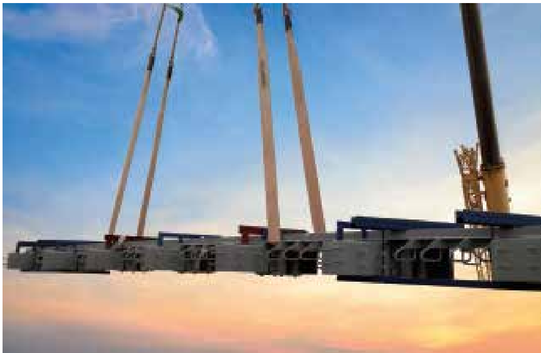
Installation of AR-EX Expansion Joints
