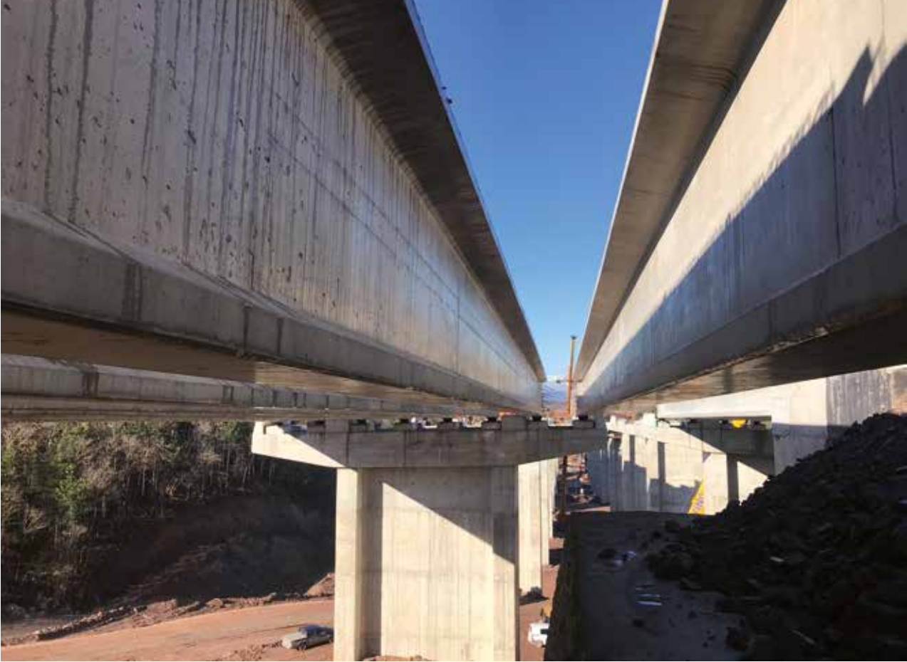
Northern Marmara Motorway – Part 5
